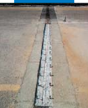
Repairing rigid joints of a highway bridge with Mapefill
