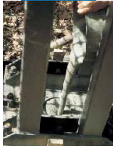
Anchoring of metallic carpentry with Mapectill
