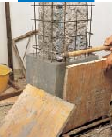
Removing wooden formwork
