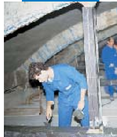
Pouring Mapegrout Hi-Flow into metal formwork
