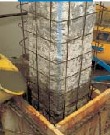
Pouring into a formwork
