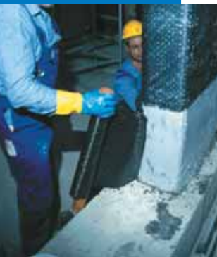
Application de Mapewrap C BI-AX
